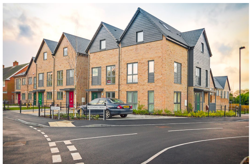
Images of the finished scheme, high quality new homes in an open and uncluttered environment
